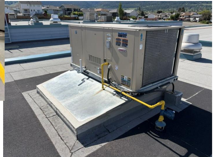
Replacement HVAC - CMS
