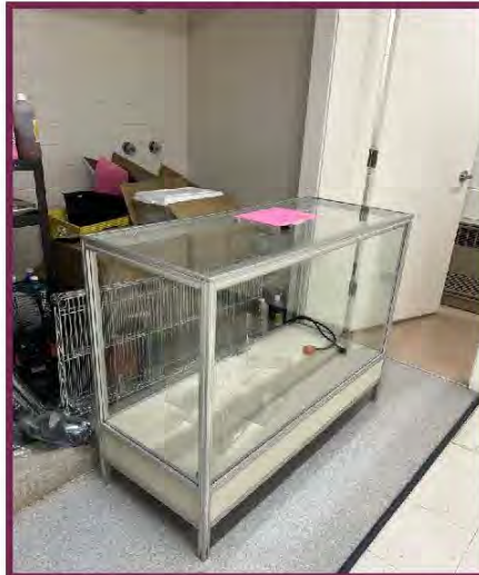
Note the tile, taps and shower heads in the former change room shower. This all will need to be removed in the remodel.
